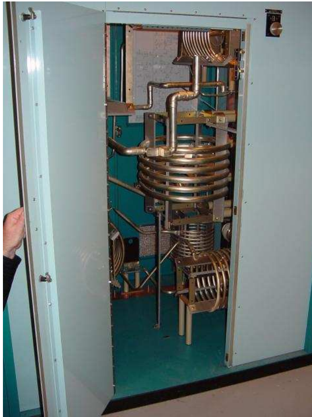
Figure 3.18: High power inductors formed from hollow tubes.
